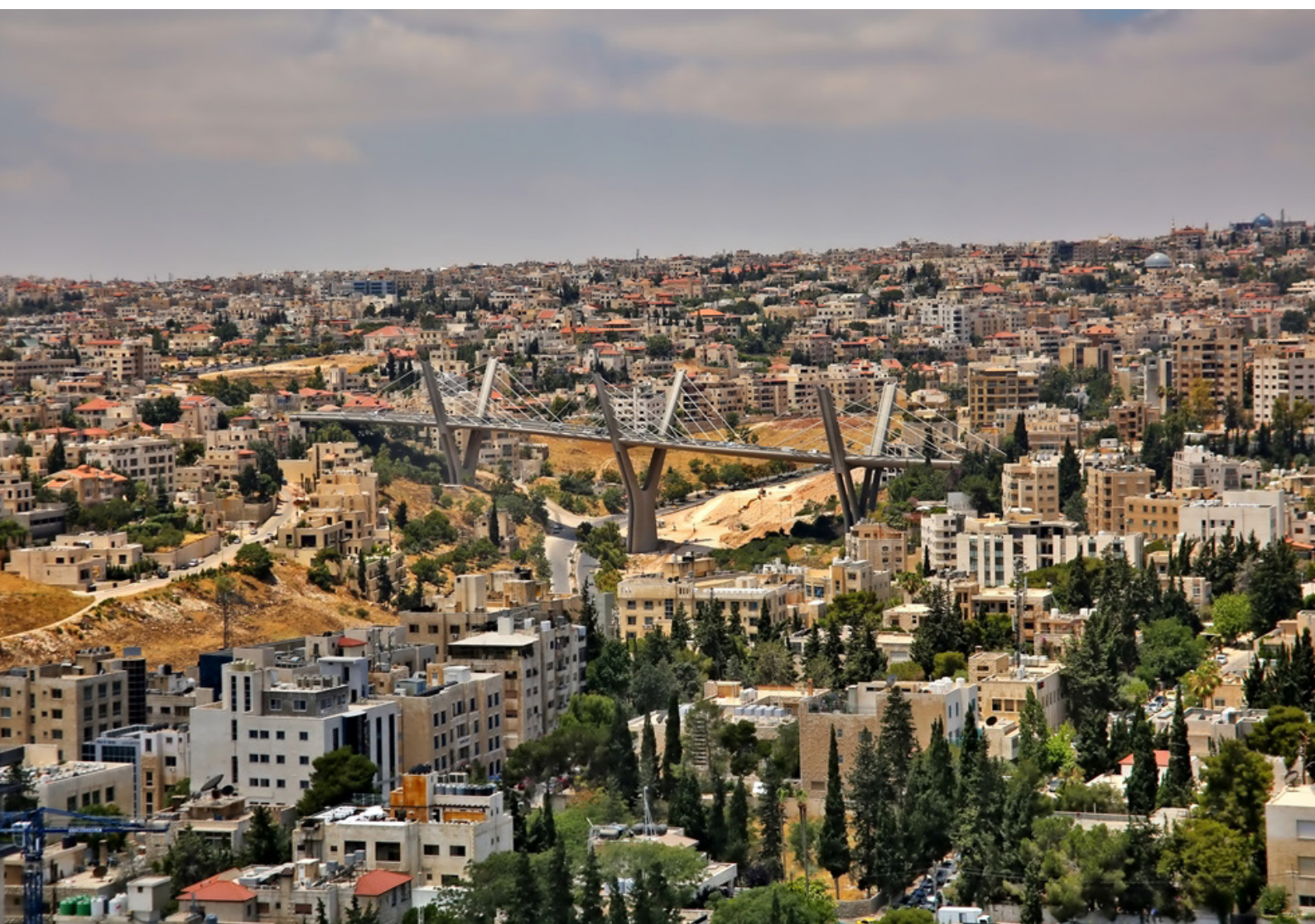
Figure 20. Abdoun Bridge, Connecting East and West Amman
